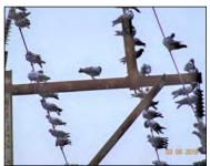
Birds are getting electrocuted during their flocking / take off from power lines in groups, specifically on top of PIN / POLYMER insulators over 33KV poles due to inter-contact of earth & live line with bird's conductive body, leading to electrocution of bird & line tripping. This problem can be avoided by using BIRD GUARDS which are designed for meeting wild life protection and extended periods of outdoor exposures along with proper fitment, insulation and easy to use.
