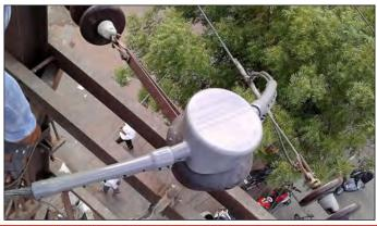
PLASTISOL bird guards exhibits various advantages in terms of customized moldability, Fire Retardance property, resistance to oil, Abrasion Resistance, Scratch resistance, adhesion, compressive strength, tensile strength, excellent gloss for good exterior appearance.
